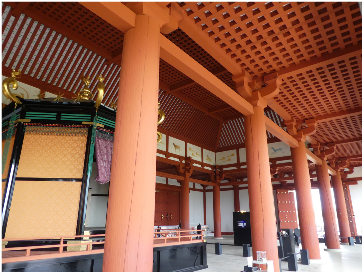
Figure 4. Pillars of the Heijō-kyū palace in Nara with smaller hinoki cypress stems bundled together. © Kizawa N.
